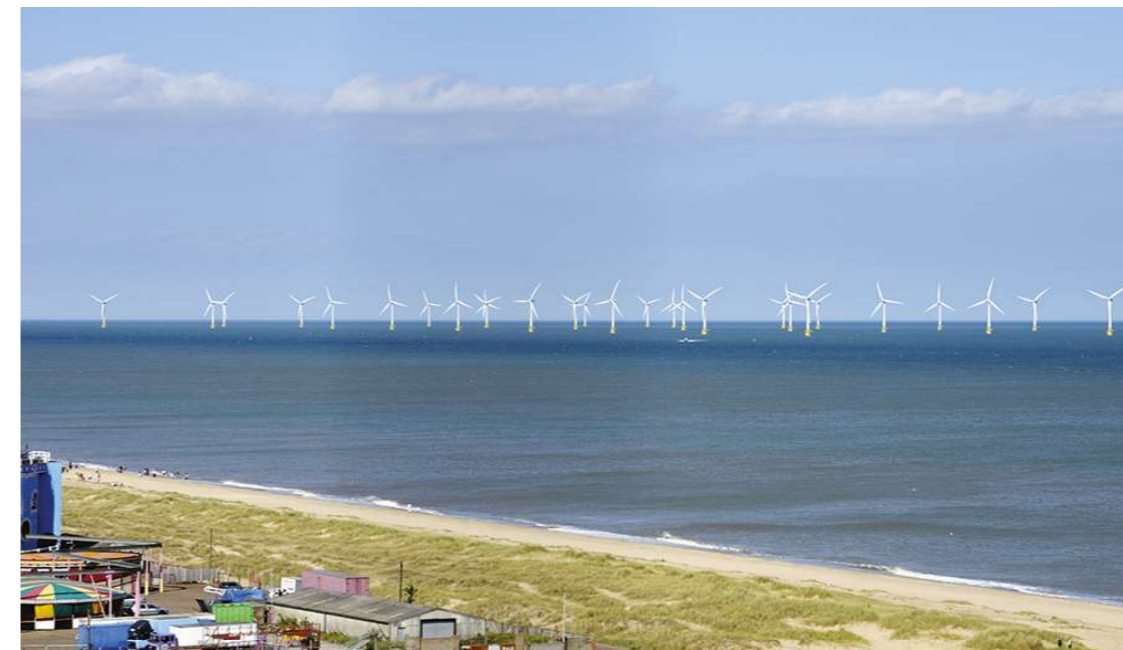
Offshore wind farm
