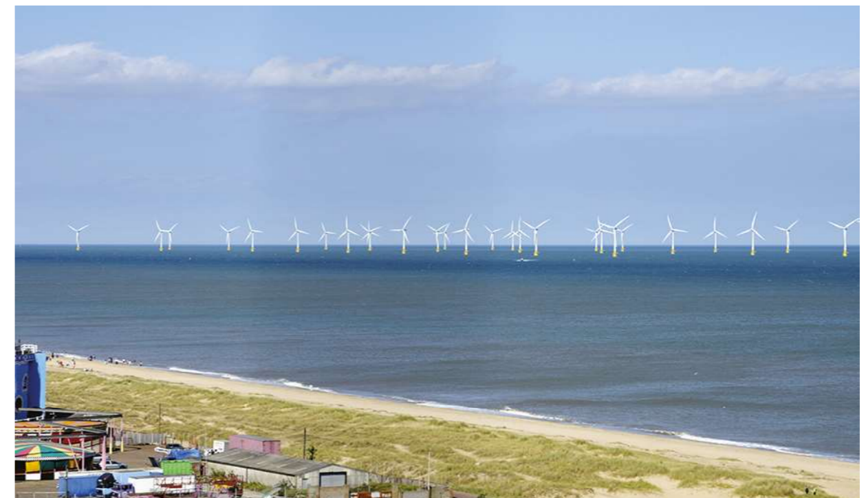
Offshore wind farm
